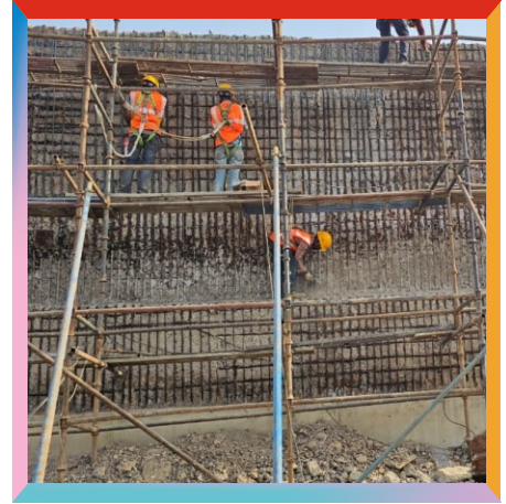
Water Tank Retrofitting
