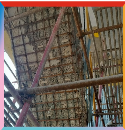
Staircase Rebar Grout
