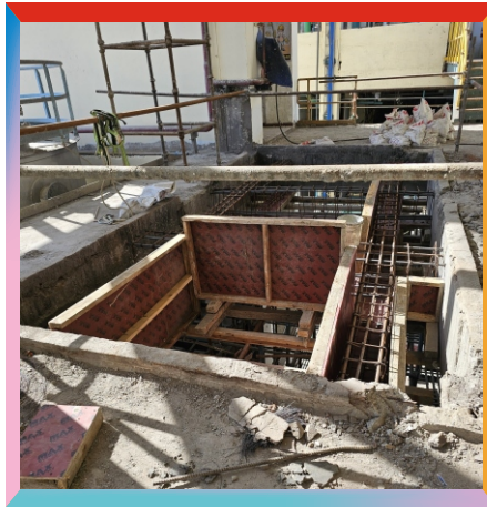
Beam Formwork
