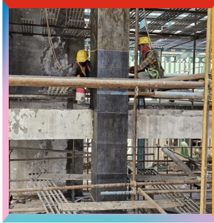
Column CFRP Work
