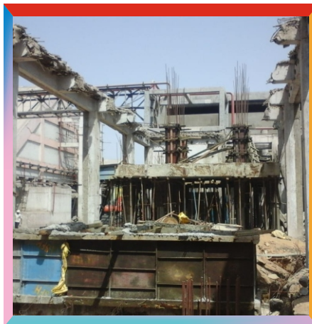
Beam Concrete Dismantle
