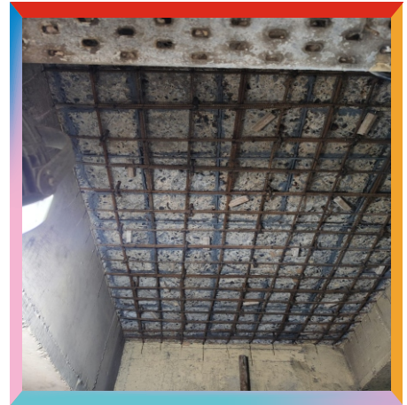
Ceiling Rebar Grout
